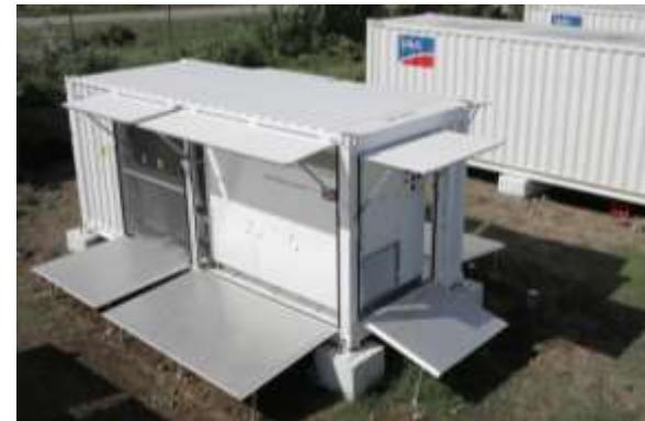
Today, solar energy covers 46% of St. Eustatius' total electricity need. Grid Forming SCS 2200 inverters allow to operate the island grid for 10.5 hours in Diesel Off-Mode operation with 100% Solar Power Fraction. In total a 5.9MWh Li-ion storage facility has been integrated for energy shifting and grid services. Thanks to the SMA Fuel Solution about 4,560 tons CO2 per year can be saved. The project has been designed, and implemented by the SMA Sunbelt Energy GmbH.
